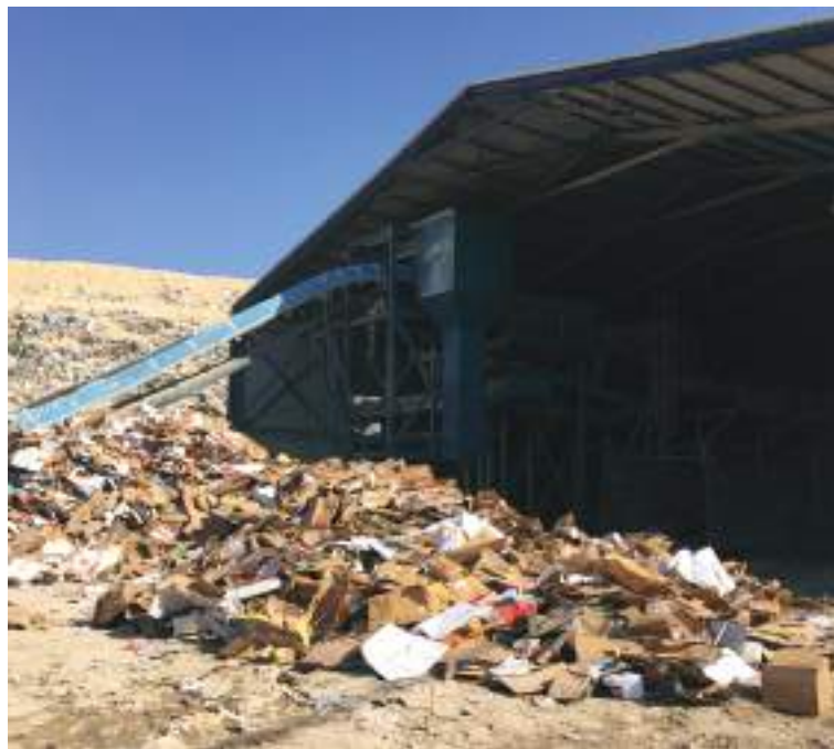
Figure 50. Carboard/paper separation area at the ZAF landfill. The sorting line in the background does not function. (V.Thöni)
