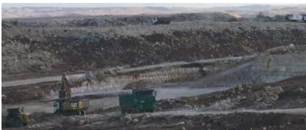
Figure 12. Al-Minya landfill, cell 5 in preparation forward and in the back cell 4 in operation. (V. Thöni)
